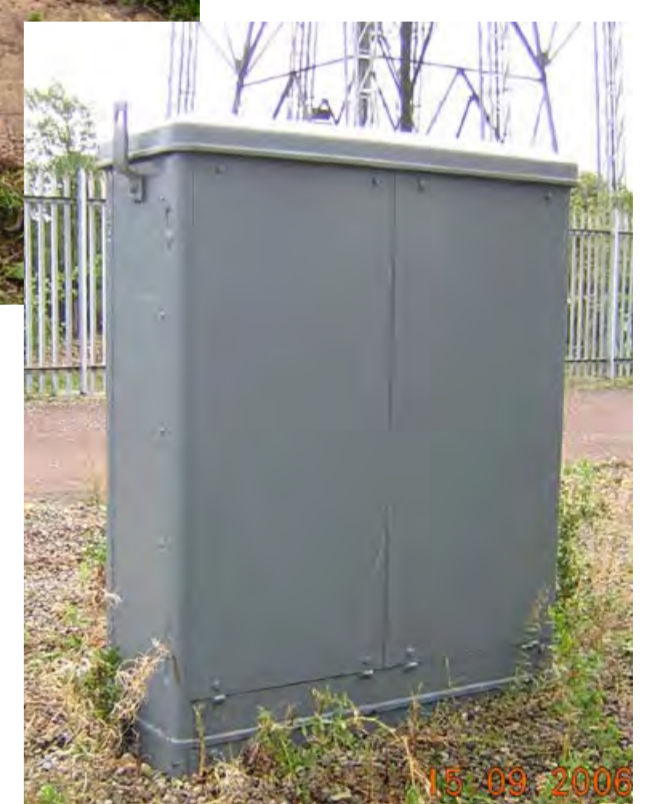
Cross bonding pit and pillar
