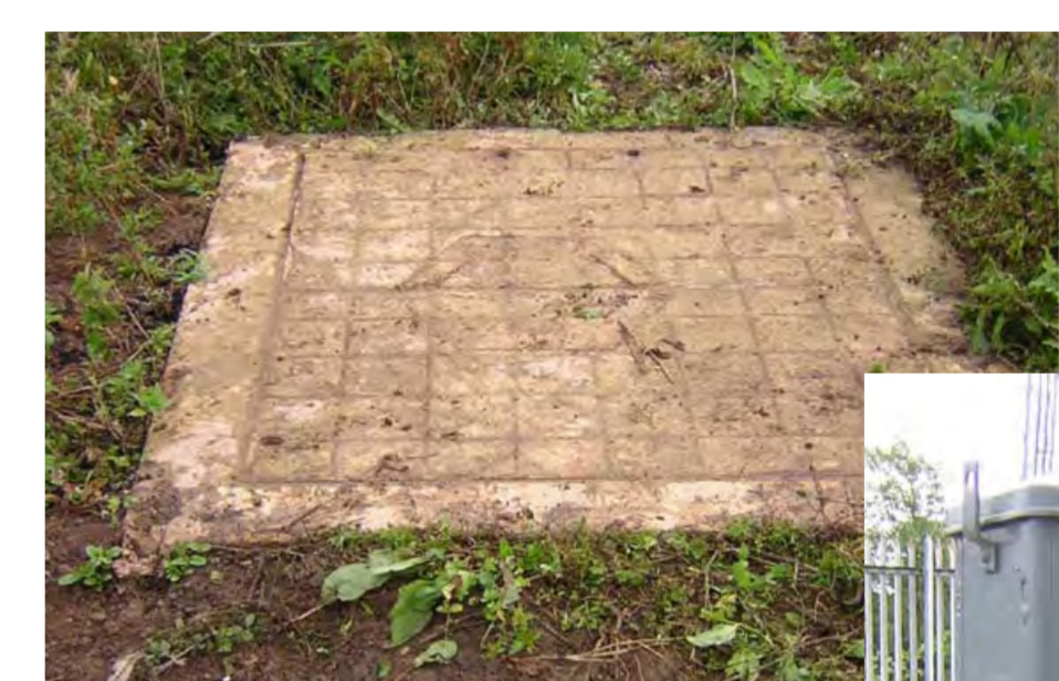
Cross bonding pit and pillar
